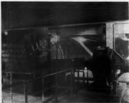
Dixie Hammer Mill in a Cement Plant
